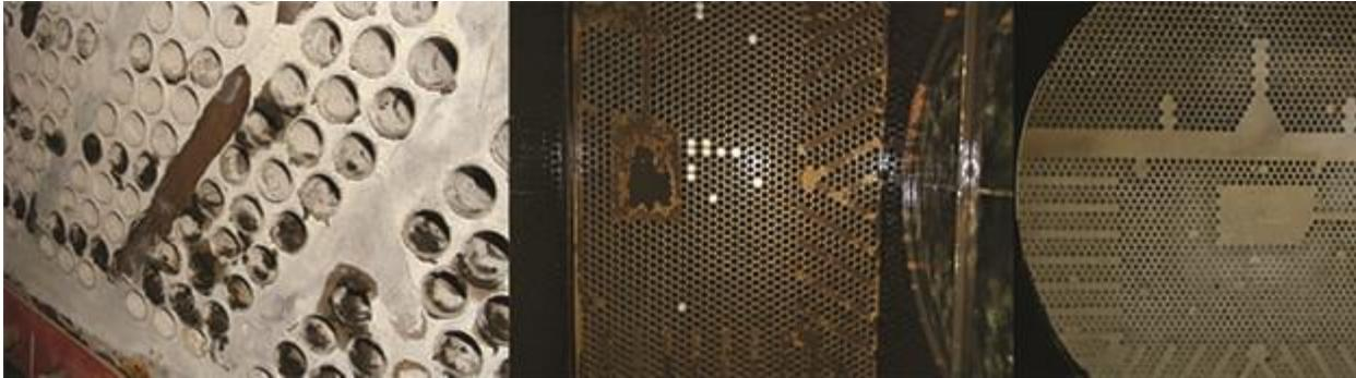
2. The image of the condenser tubes on the left was taken before installation of the Flow-Tech treatment system. The center and right-side images show a dramatic decrease in fouling after the Flow-Tech system was operated. Courtesy: Flow-Tech Systems
