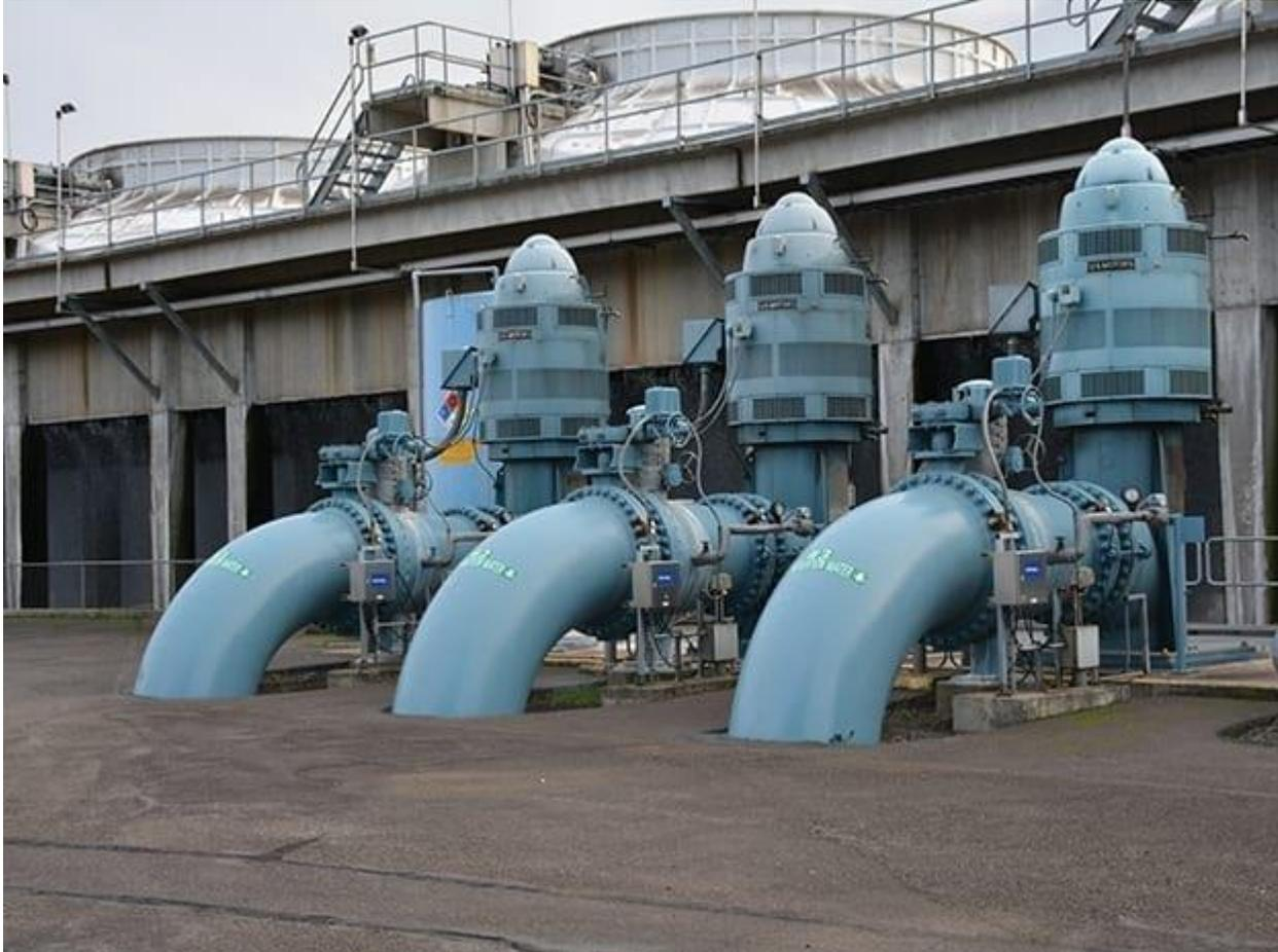
*1. Flow-Tech electronic treatment technology is installed through a non-invasive process. System components are shown here mounted on flanges on the discharge of circulating water pumps. Courtesy: Flow-Tech Systems*
